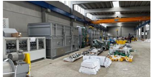
Oggiono plant - Installation of the new hardening and tempering line
